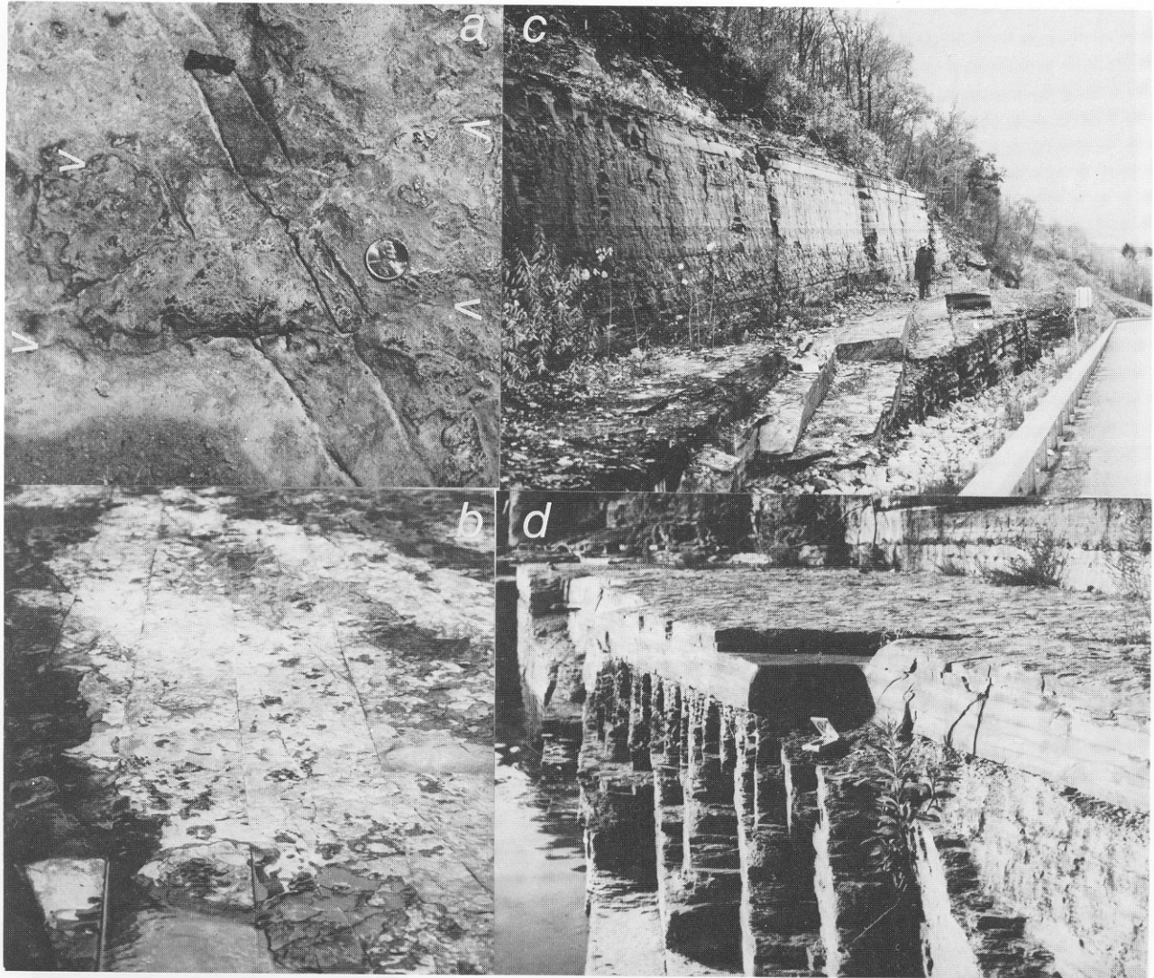
Fig. 6. (a) Set Ib joints within the Tully Limestone at Ludlowville Falls, New York where a later Main Phase Alleghanian cleavage cuts the joints (arrows). Coin is 1.8 cm in diameter. (b) Cross-fold joints within the Genesee Shale Formation of the Genesee Group at Taughannock Falls State Park, New York. Later joints are seen curving into earlier joints with the later joints being counterclockwise from the earlier joints. These joints are believed to belong to the same set although the variation in orientation is anomalously high. The joint spacing is about 1 m. (c) Cross-fold joints along route 414 at Watkins Glen, New York (after Bahat & Engelder 1984). The early joints formed within the thinner siltstone beds at the man's feet while the later joints formed within the thicker shale beds next to the man. The earlier joints are counterclockwise from the later joints. (d) Cross-fold joints within the upper portion of the Genesee Group at Taughannock Falls State Park, New York. The early joint (set Ib) within the thin siltstone bed is counter-clockwise from the later joints (set Ia) with the underlying shales. The siltstone bed is 19 cm thick.
